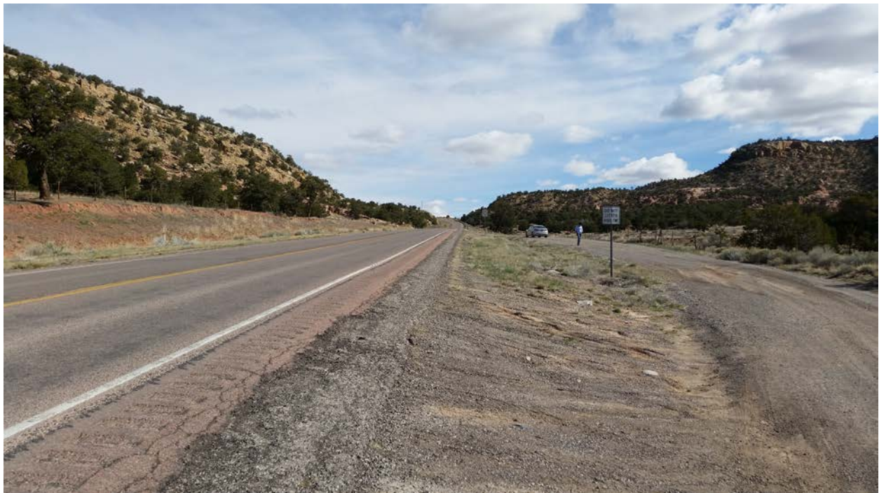
Figure 4-9 Approach To San Antonio Hill From The South
